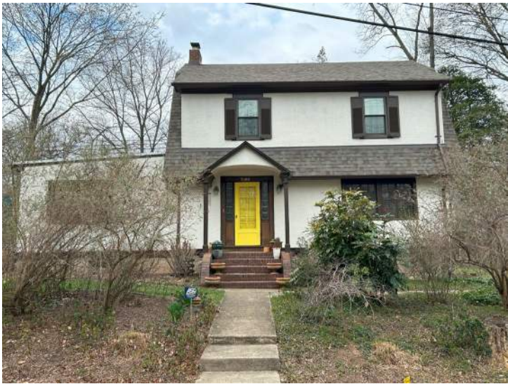
West Side – Outside of Historic District
